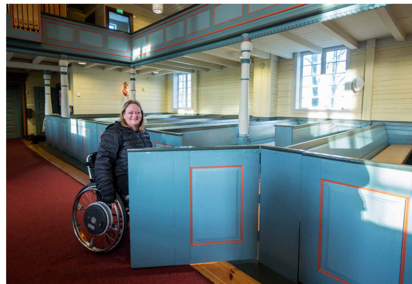
WIDE ENOUGH: The door was merged with the side panel. That way the opening fits Sissel Løchen - without interfering with the visual expression. (Photo: Fredrik Naumann)
