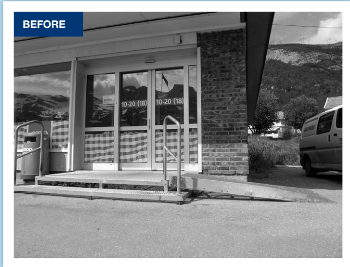
BEFORE: Two steps and a ramp to access the shop.
