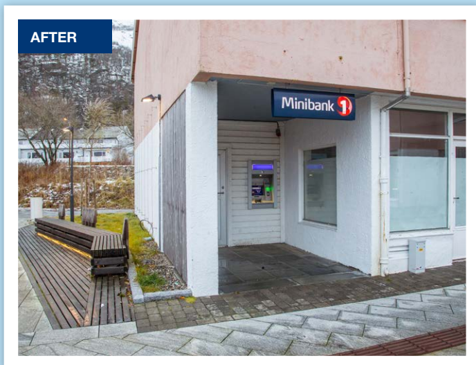
AFTER: Step free access to the cash machine, which is also given a protective wind screen.
