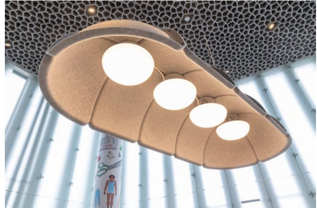
TWO IN ONE: Soundproofing and lighting in one. The ceiling also has a soundproofing design.
