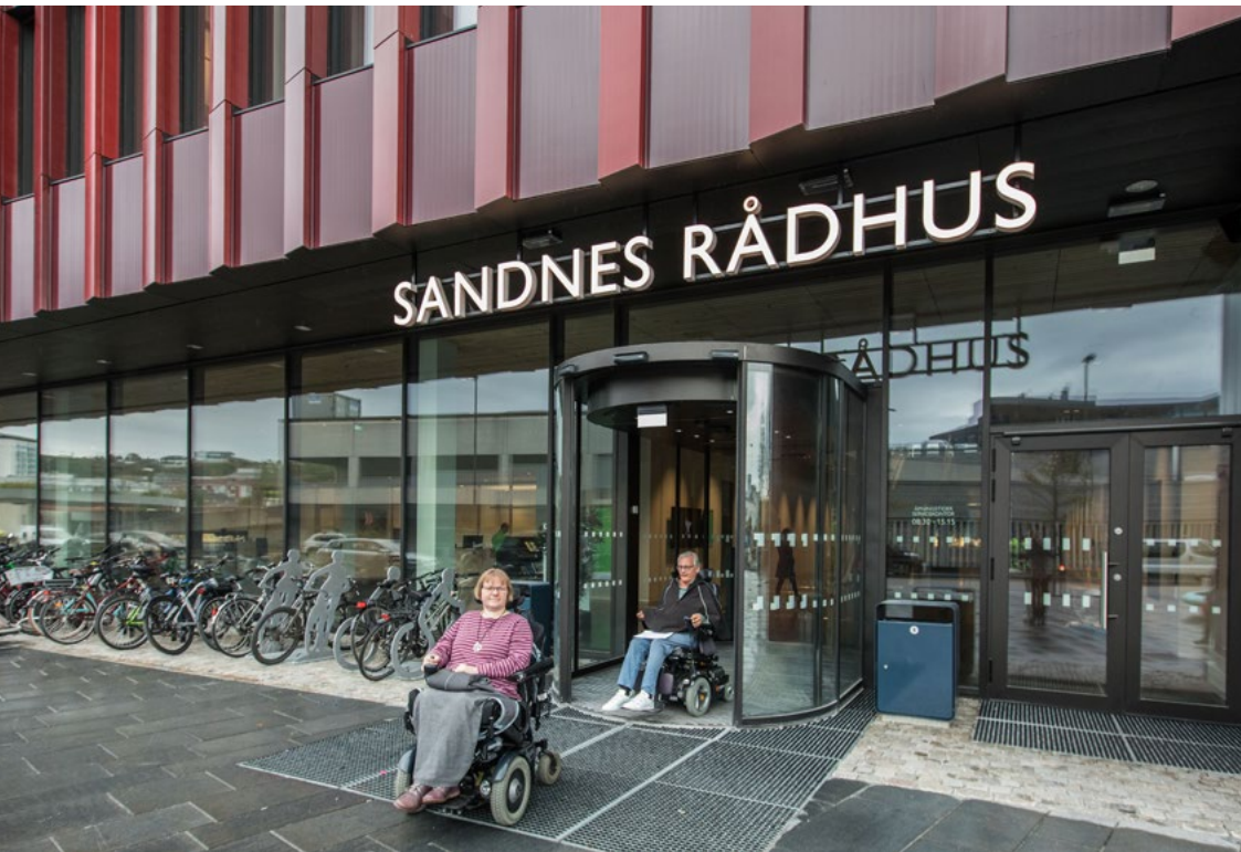
MAIN ENTRANCE FOR ALL: Sliding doors in a ‘vestibule’ – and with contrasting colours – work for all users, whether they have a visual impairment, walking difficulties or use wheels.
